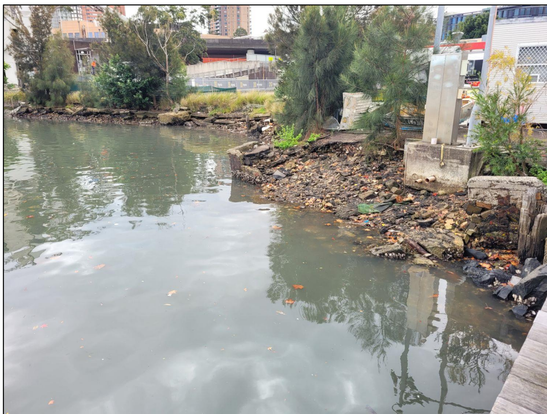
Plate 1 – Foreshore area north of jetty at the existing Fishmarkets
